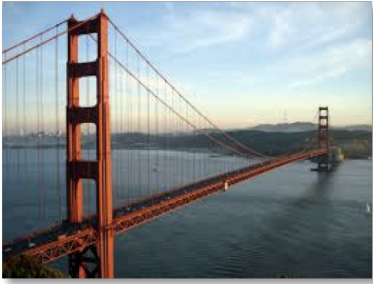
Golden Gate bridge (San Francisco)
